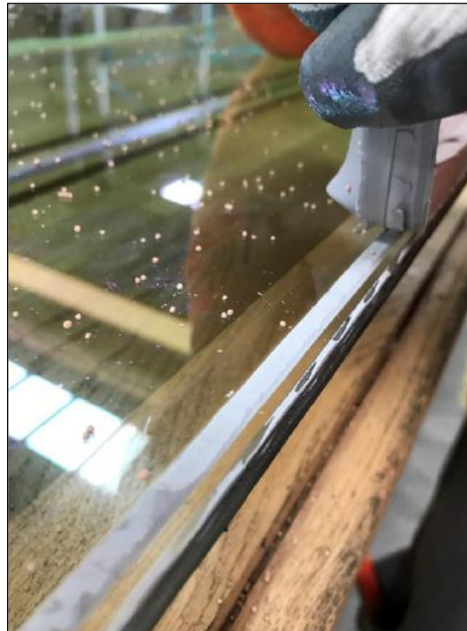
Figure 36: Adhesive failure, deglazing test negative
