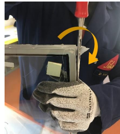
Figure 41: Pressing the chisel downwards
