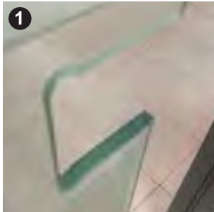
1) Carefully clean the glass near the cut out.
