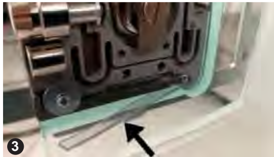
3) Insert the 1 mm PVC spacer to remove the possible space between the cutout and the plate. Cut the excess part.
